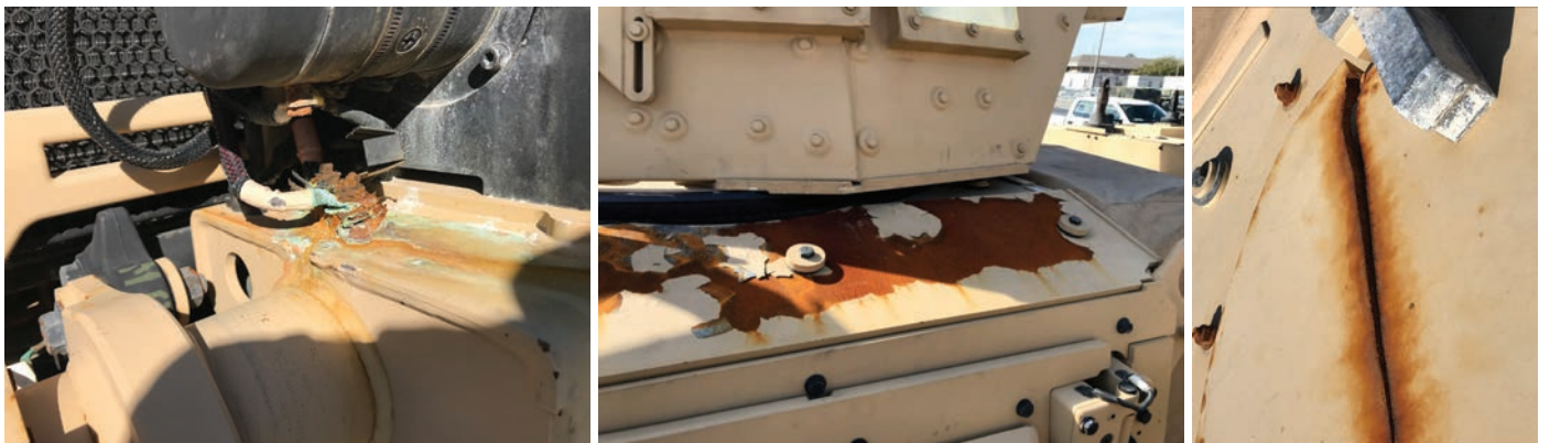
Figure 2. Corroded electrical connections and paint failure leading to corrosion. (Figure provided by Eric Brown.)
