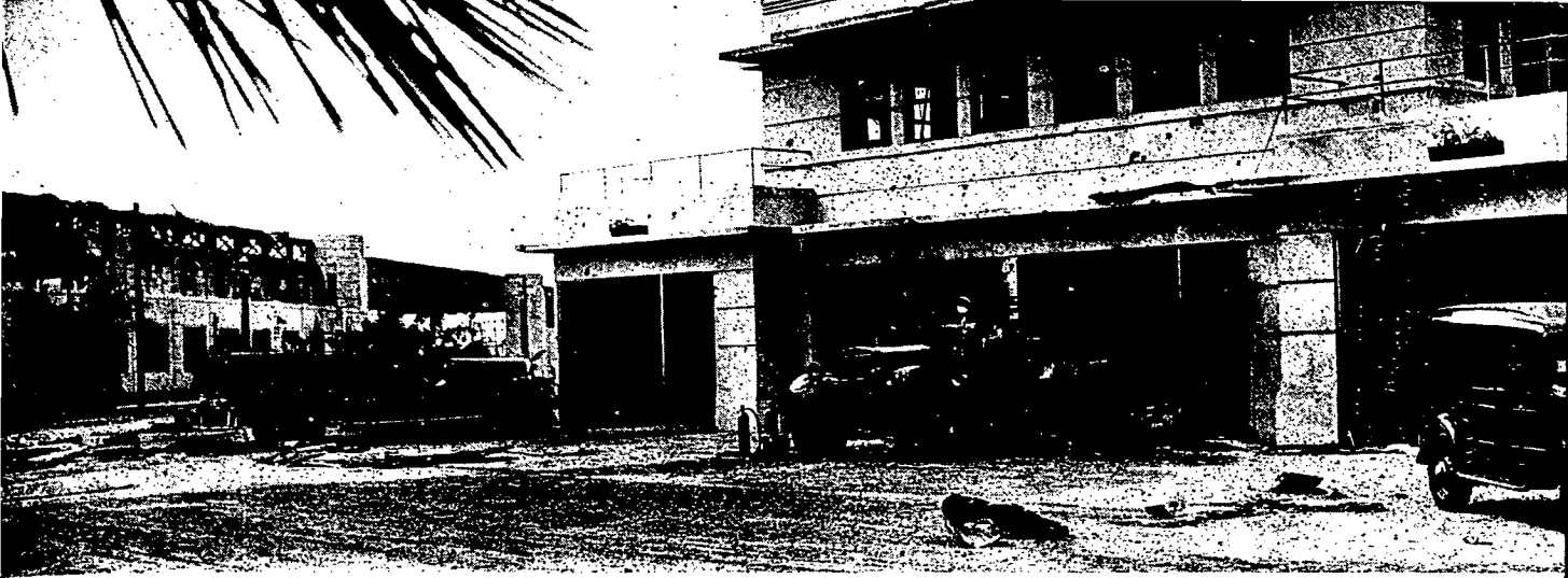
FIRE STATION at Hickam Field razed by fire and machine guns. Fire trucks were badly burned and intersection seriously damaged.
