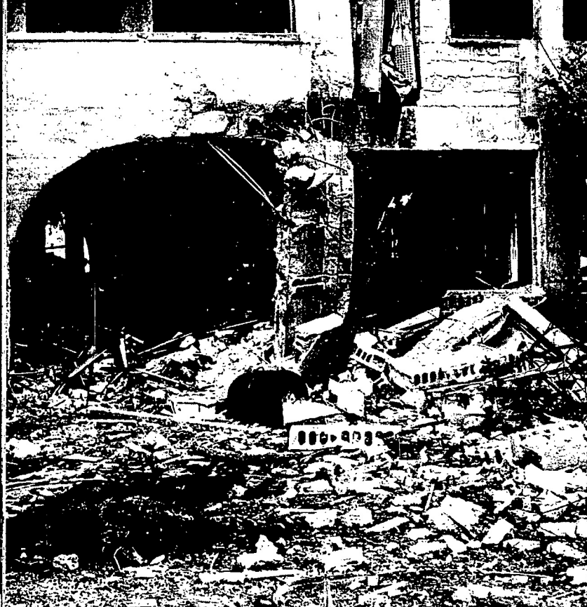
FORCE OF EXPLOSION inside barracks at Wheeler Field blew out sides of building. Concussion wrenched lockers open, strewing clothes amidst the wreckage. Sudden attack caught many men in the barracks when the first wave struck.
