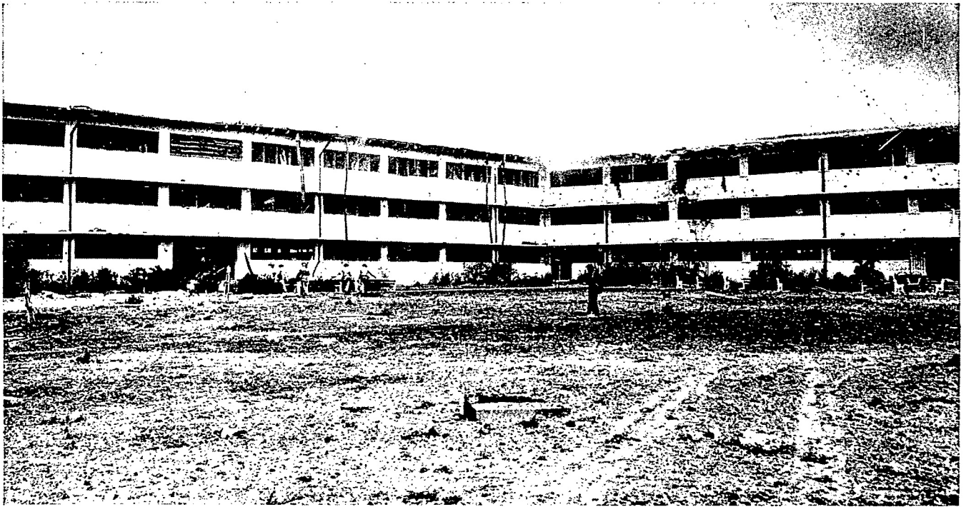
DIRECT HITS WERE MADE in many places in the crowded barracks at Hickam Field. Soldiers rushed hand extinguishers to the blazes started in the new barracks.
