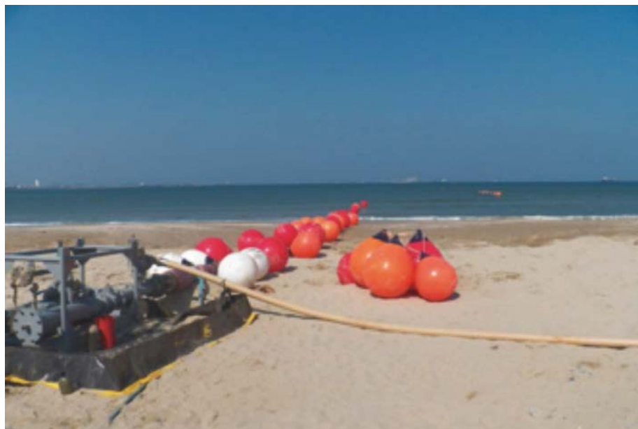
MV Wheeler Offshore Petroleum Distribution System (OPDS) connection to the Beach Terminal Unit (MV Wheeler in the background). (Photo by 3D MEB COMSTRAT.)
