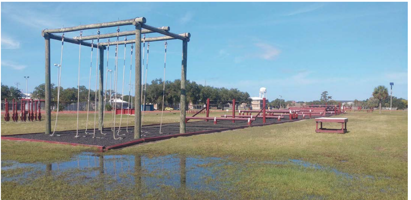
Localized flooding around 4th Battalion obstacle course. (Photo by Capt Brandon Barnes.)
