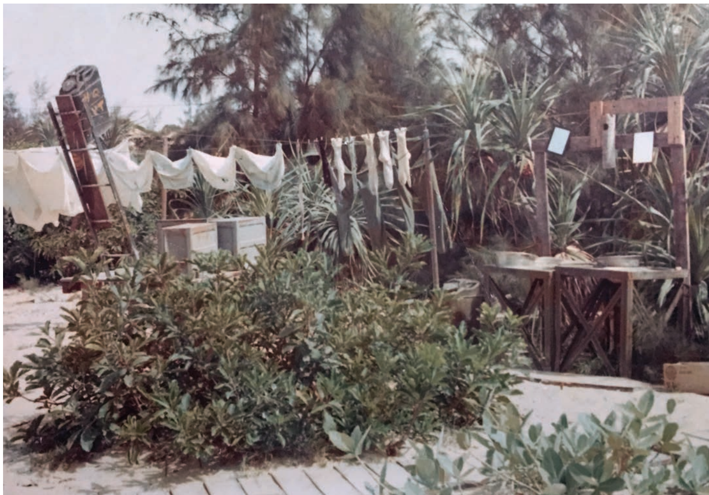
Thanks to typical Marine ingenuity, Marines at Chu Lai constructed a shower made from a 5-gallon water can on a rotating board with wash rack for clothes, two sinks made from pans, and shaving mirrors.
