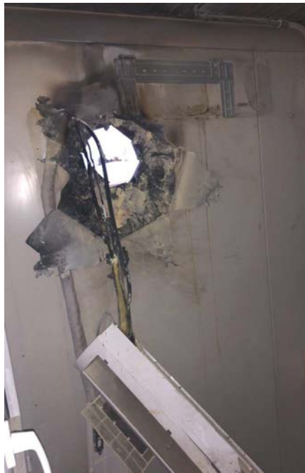
A Rocket Propelled Grenade hole in the CONEX box used as living quarters for contract workers at Camp Shorab.
