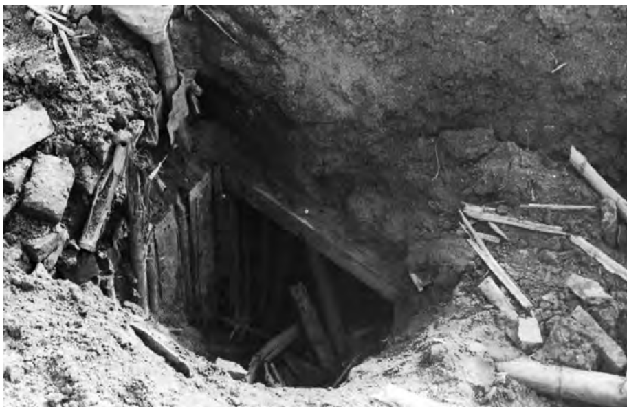
Above: Deep underground and connected by tunnels, bunkers found in the Hook concealed fire ports looking out over the open ground through which Marines passed.
