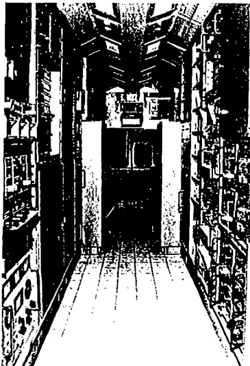
External and Internal Views of Tactical Air Operations Module (TAOM): Figure 5-7 Photos courtesy of Litton Data Systems, Van Nuys, California
